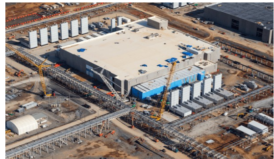
An under-construction data centre in Virginia, US.
